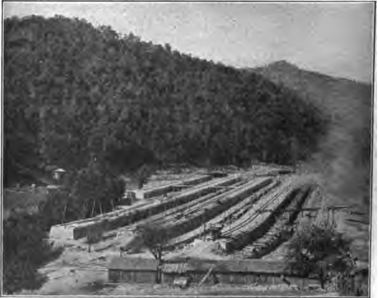
FIG. 98.—The little mine car brings the coal to the wasteful beehive ovens and the box car carries away the coke. Western Pennsylvania.
